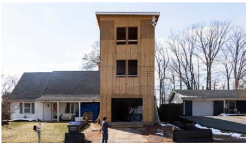
Large addition to existing home to allow additional dwelling units
