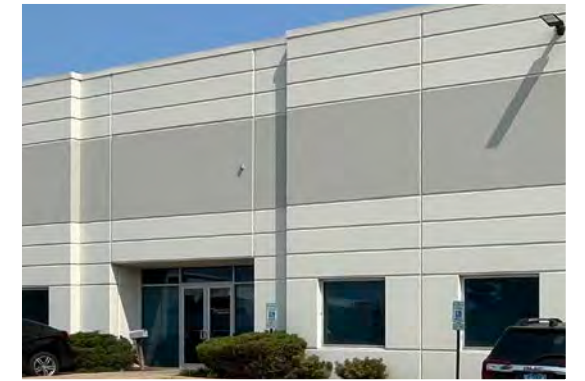
EXTERIOR INSULATION AND FINISH SYSTEMS (EIFS)
